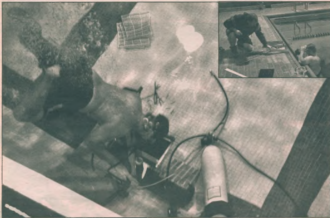
Chad Seidler is starting the correction of the non-compliant pool drain at the Vadalabene Center's indoor pool Wednesday. Inset: Ray Gallup (left) and Chad Seidler (right) continue the pool drain update.
